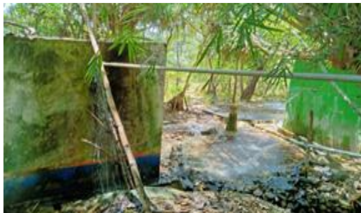
Figure 3, there are two (2) water reservoirs
